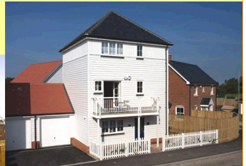
Whitesands, Camber Phase 2 – 36 timber framed houses on behalf of Southern Heritage
